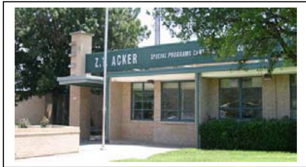
Acker Office Complex 7159 Hickory St. Frisco, Texas 75034
